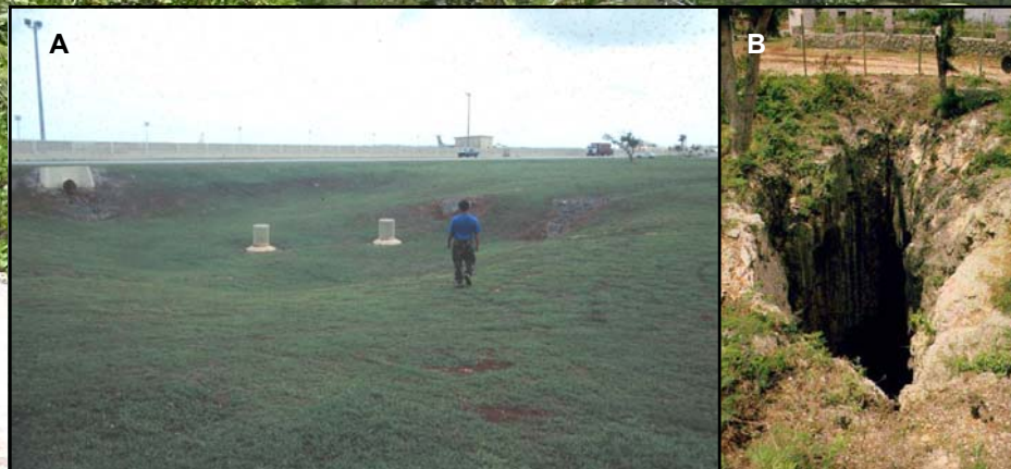
Figure 5: A) Injection wells acting as artificial vadose fast flow routes at Anderson Air Force Base, northern Guam. The wells deliver runoff from the runway directly to the deep aquifer. B) Natural vertical shaft, acting as a 40 m deep vadose fast flow route, Amantes Point, Guam.
