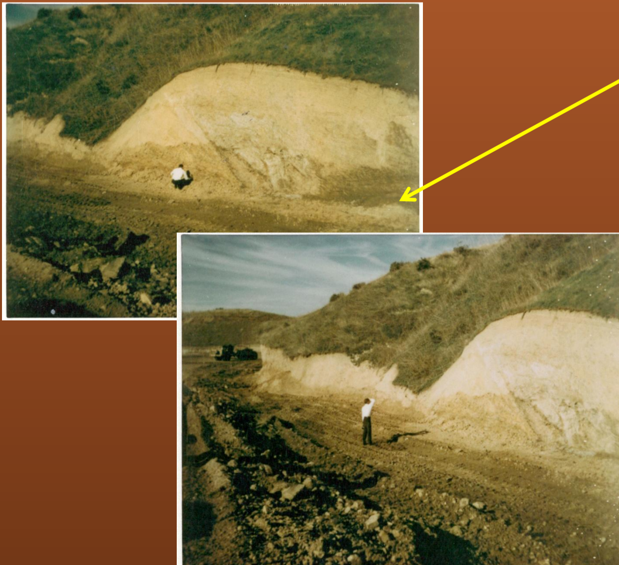
Photos taken in 1970 during initial canyon cleanout operations prior to Tonner Canyon fill placement. Views looking west at northeast-dipping Whittier Fault. Photos courtesy of Robert E. Tepel
