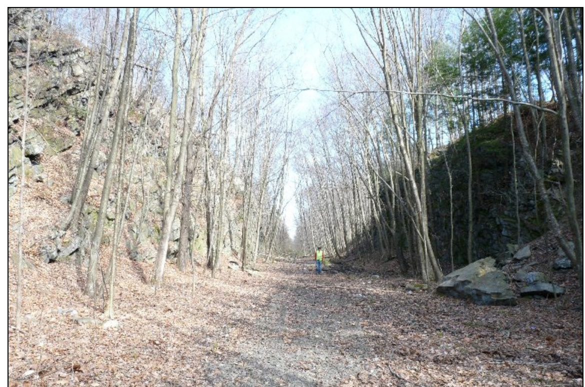
Abandoned cut through Shawangunk Mountain in the wind gap at Otisville, looking east (GPS 41° 28' 32.4"N/74° 33' 05.9"W). The cut is 0.5 mi south of the later tunnel and several hundred feet higher in elevation. The beds exposed are northwest-dipping (~30°) quartzitic conglomerate and sandstone of the Shawangunk Formation, the unconformable contact with the Martinsburg Formation being exposed at the east end of the cut.
