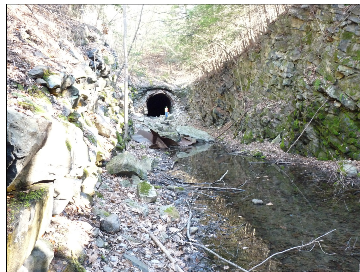
Long rock-cut in Shawangunk quartzite and quartz conglomerate in the approach to the northwest portal of the High View tunnel.
