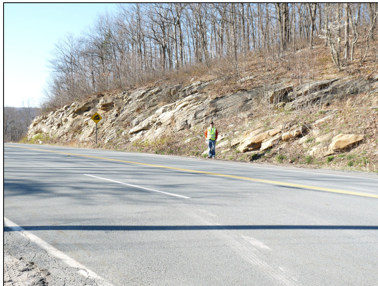
Cut in Shawangunk Formation along old NY Route 17, a few hundred yards north-northwest of the northwest portal of the High View Tunnel. Bedding dips to the northwest.
