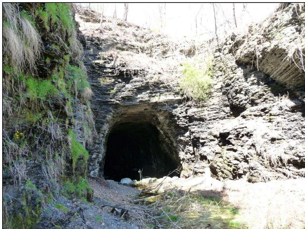
Southeast portal of the High View tunnel near the former High View Station on the east flank of Shawangunk Mountain (GPS 41°33' 30.3"N/74° 27' 30.6"W). Bedding in the Martinsburg shale here strikes N65E and dips 14°NW on the west limb of a minor anticlinal fold.
