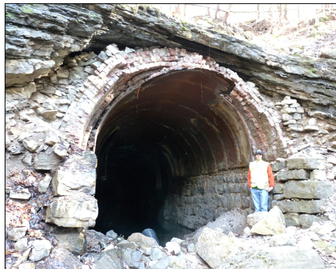
Northwest portal of the abandoned O&W High View tunnel about 0.8 mi east-southeast of Wurtsboro (GPS 41° 34' 00.0"N/74° 28' 05.7"). The Shawangunk conglomerate here strikes N33E and dips 26° NW. Note the iron, brick, and crushed stone (from interior out) linings of the tunnel exposed in a botched attempt to shorten the tunnel sometime in the past.
