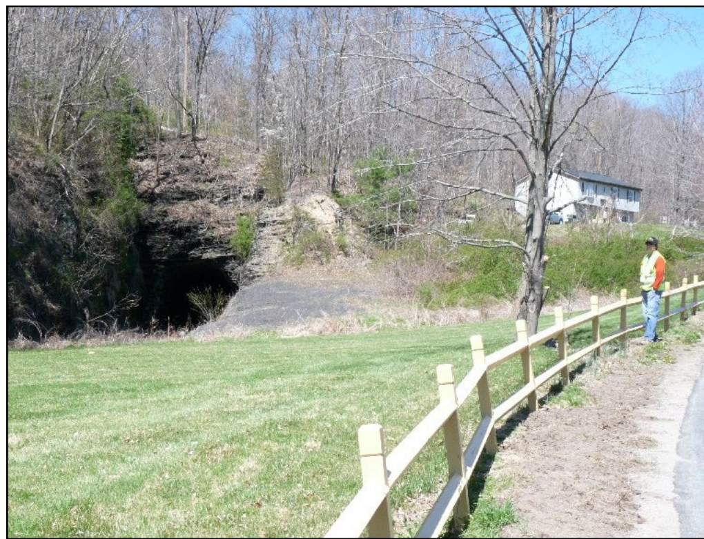
Southeast portal of the abandoned O&W tunnel at High View (GPS ~41° 33' 30.3"N/74° 27' 30.6"W). Bedding in the Martinsburg shale and sandstone in the immediate vicinity of the portal is very gently west dipping.
