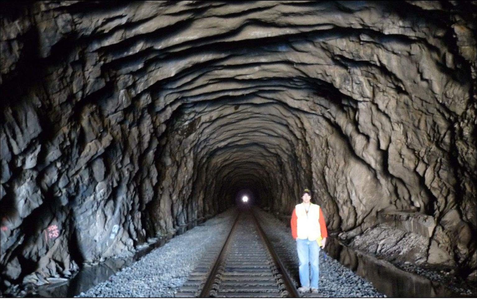
Unlined west part of the Erie Railroad tunnel at Otisville. The Shawangunk conglomerate here forms a ragged, but solid, arch that does not require lining.
