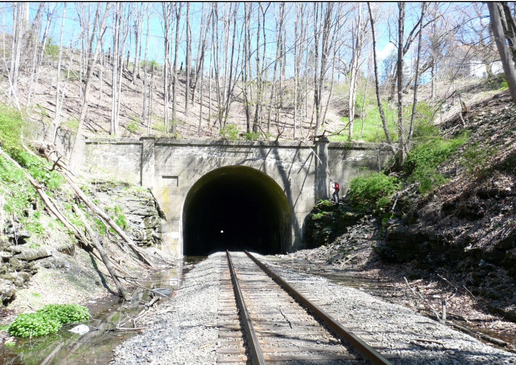
East portal of Erie Railroad tunnel at Otisville (GPS 41° 28' 25.1" N / 74° 32' 13.2" W). Intensely deformed Martinsburg shale and sandstone are exposed on both sides of the cut leading into the tunnel.
