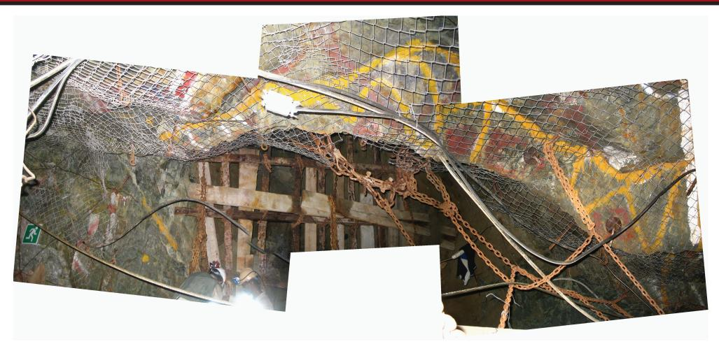
Fencing erected to stabilize a fault in TauTona mine in a region where the tunnel collapsed during a M1.8 earthquake on 12 December, 2004. (Photo provided by V. Heesakkers and Z. Reches)
