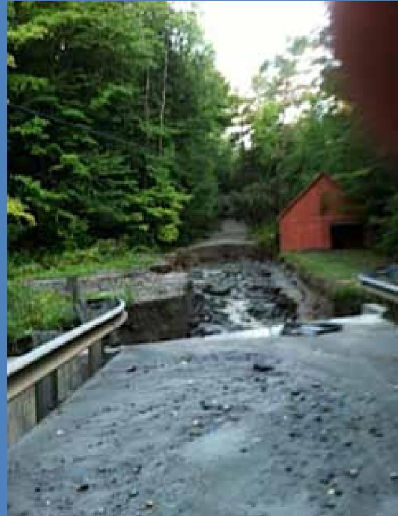
Woody debris on bar and road damage, looking downstream on White River in Stockbridge. Long sections of Vt. Rt. 107 were destroyed. In addition to fluvial erosion, numerous failures occurred on the slopes above the highway.
