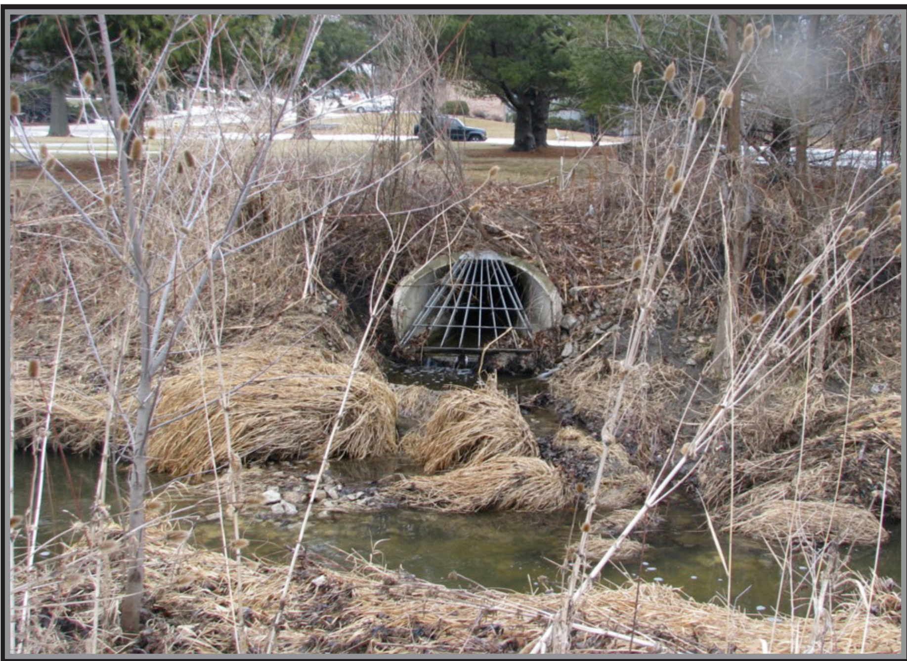
Figure 2. A storm sewer outlet to Sugar Creek from a residential storm sewer shed
