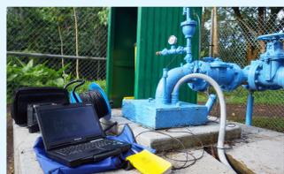
Figure 10: Offline production well. Static water levels were used for model calibration.
