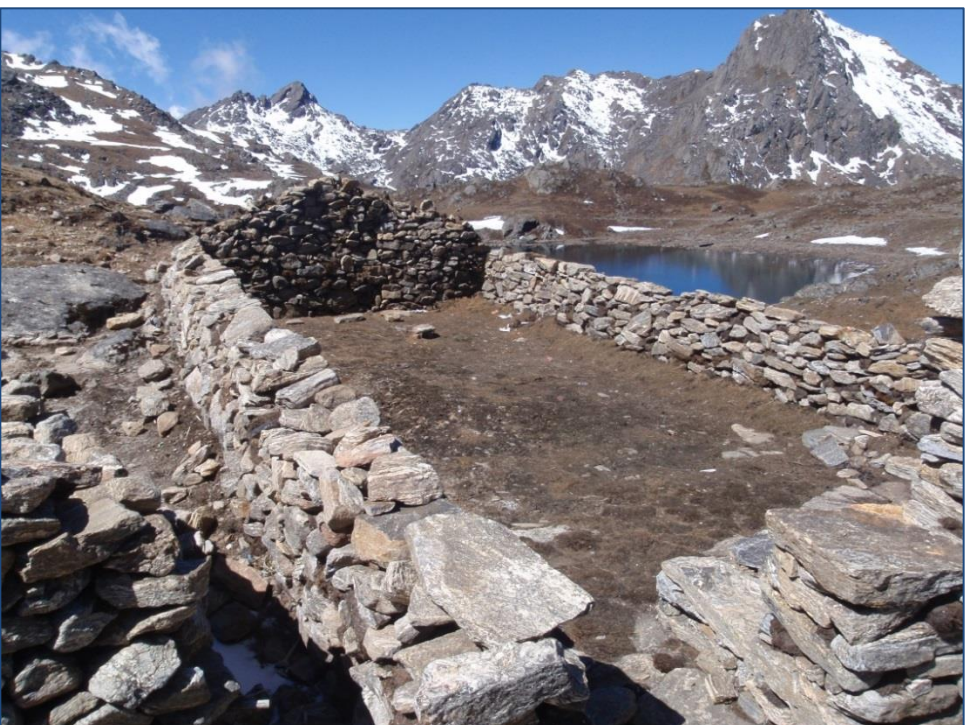
Fig. 14 Roofless stone huts (called kharkas) are common between Shin Gumpa and Phedi, especially in the vicinity of Gosaikund (see Fig. 3). Many of the stones are cut, although they lack the elaborate carvings found on the mani walls between Ghoratabela and Kyanjin Gumpa (see Fig. 4). Although the roofless stone huts are rebuilt annually, there is probably a foundation that is rarely rebuilt.
