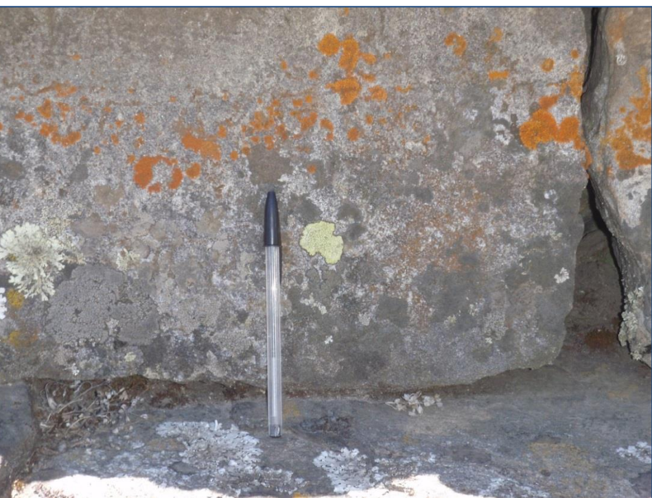
Fig. 7 The age (time since last cleaning) of each mani wall was estimated using the maximum lichen size found on each mani wall.
