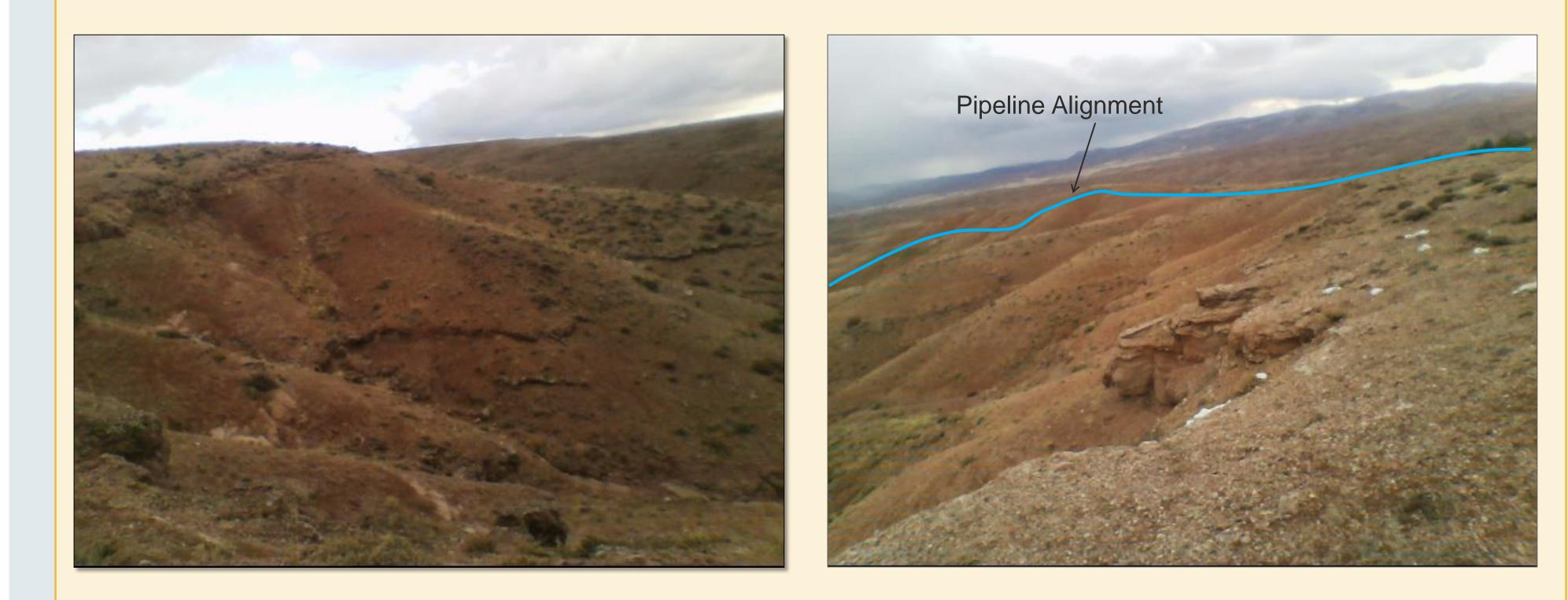
**ENGINEERING RECOMMENDATIONS.** Pipeline typically is routed along ridge crests in such terrain, so negligible likelihood of pipeline rupture from continuing erosion. However, route inspection is required during operation to identify and remediate erosion/gullying before creating unsupported pipeline spans.
