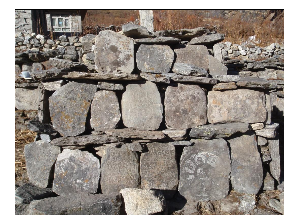
Fig. 12 Although Mani Wall No. 44 had no apparent damage, the largest lichen in 2015 was 38.28 mm, although no lichens were present in 2009 or 2014. The most likely explanation is that the mani wall had already been reconstructed in such a way that a formerly interior block was placed on the exterior of the mani wall. The mani wall was in the village of Mundu (Fig. 5), which was inhabited at the time of the 2015 fieldwork (note house in background). The three reconstructed mani walls (Nos. 44, 53, 54) are within 195 m of one another.
