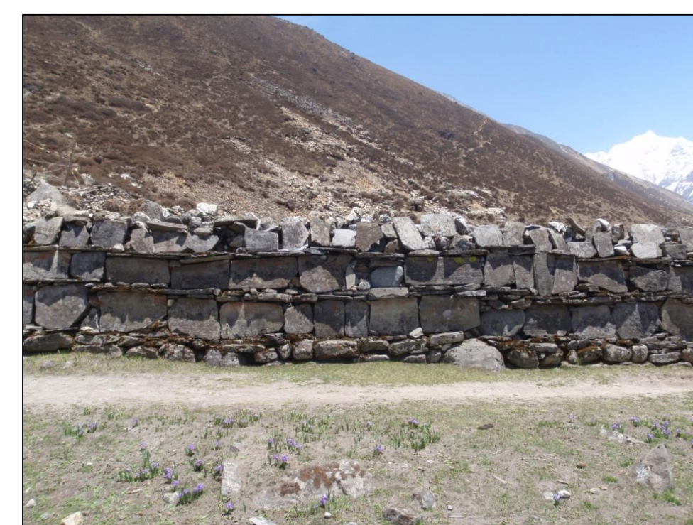
Fig. 1 Buddhist sacred walls, called mani walls, are common in Langtang Valley (Nepal Himalaya) and especially between the site of the former Langtang Village and Kyanjin Gumpa. This mani wall is adjacent to the monastery in Kyanjin Gumpa (Mani Wall No. 80). The mani wall suffered no apparent damage from the 2015 Gorkha earthquake, although the monastery was heavily damaged.
