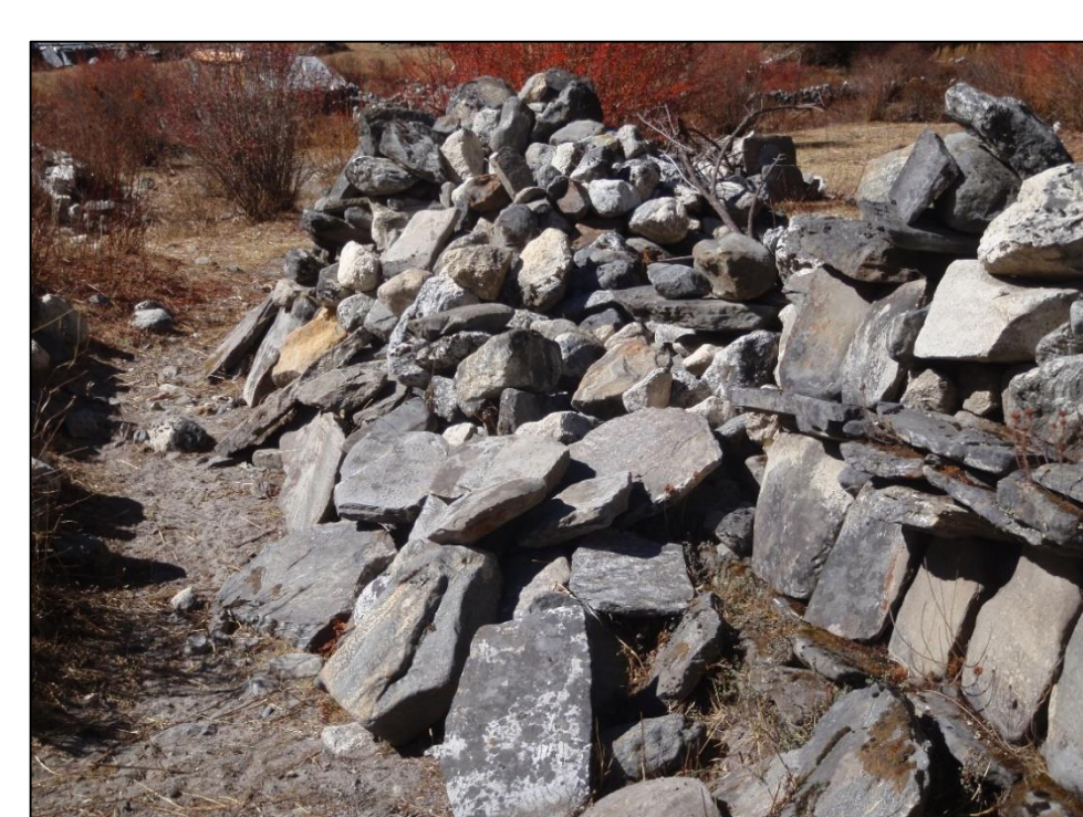
Fig. 6 Mani Wall No. 64 was classified as "severely damaged" because it was not obvious how to reassemble the fallen blocks. The largest lichen found in 2015 (49.05 mm) was much larger than the largest lichen found in 2014 (22.82 mm) and was not the same lichen. Most likely, the earthquake damage exposed a larger lichen on an interior block.
