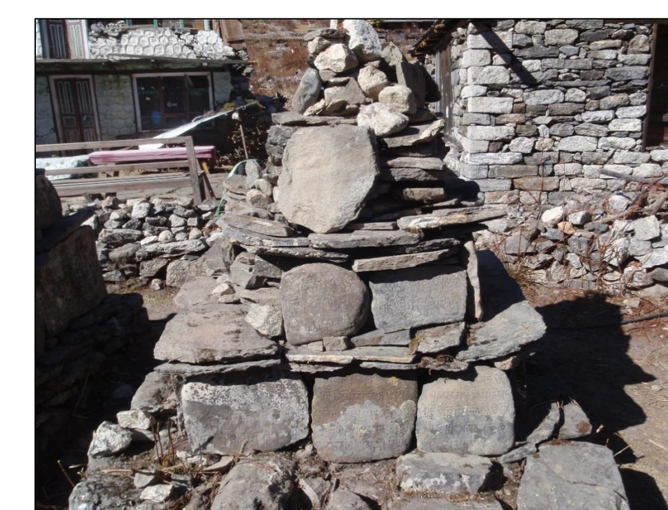
Fig. 10 Although Mani Wall No. 53 had no apparent damage, the largest lichen in 2015 was 43.42 mm, although no lichens were present in 2009 or 2014. The most likely explanation is that the mani wall had already been reconstructed in such a way that a formerly interior block was placed on the exterior of the mani wall. The mani wall was in the village of Mundu (Fig. 5), which was inhabited at the time of the 2015 fieldwork (note house in background).
