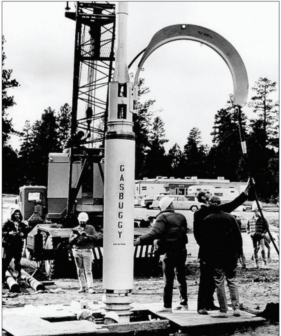
Figure 14. Gasbuggy nuclear device (13 ft long, 18 in. in diameter) being lowered into emplacement hole GB-E ([www.lanl.gov/newsroom/photo/history.php](http://www.lanl.gov/newsroom/photo/history.php); history, gasbuggy device).
