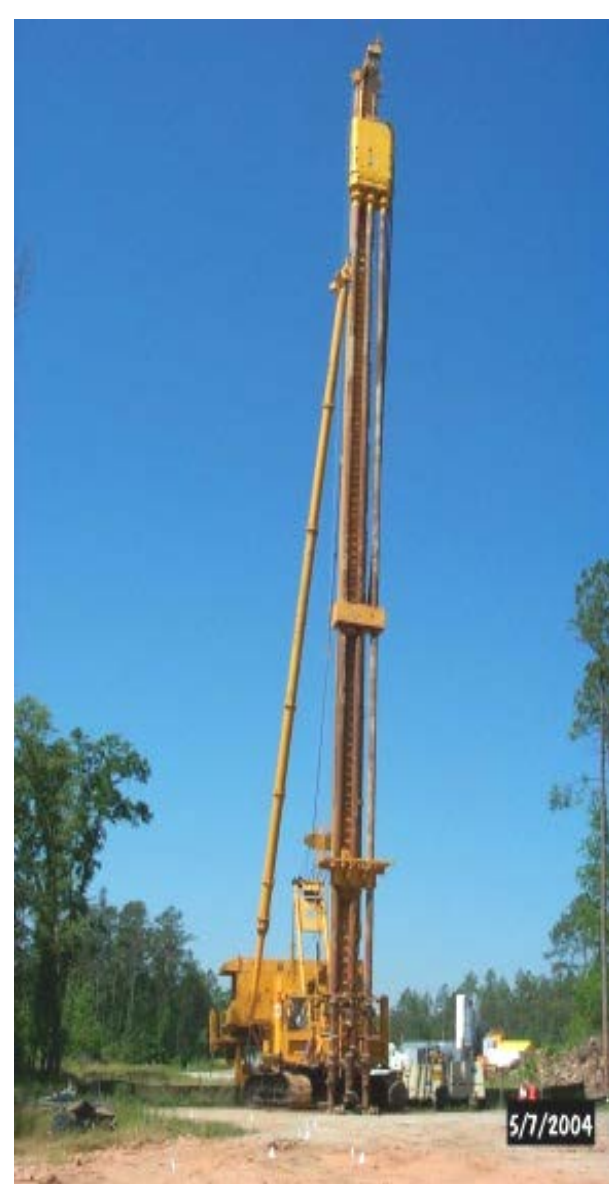
Slurry wall drilling and conceptual design of funnel & gate
