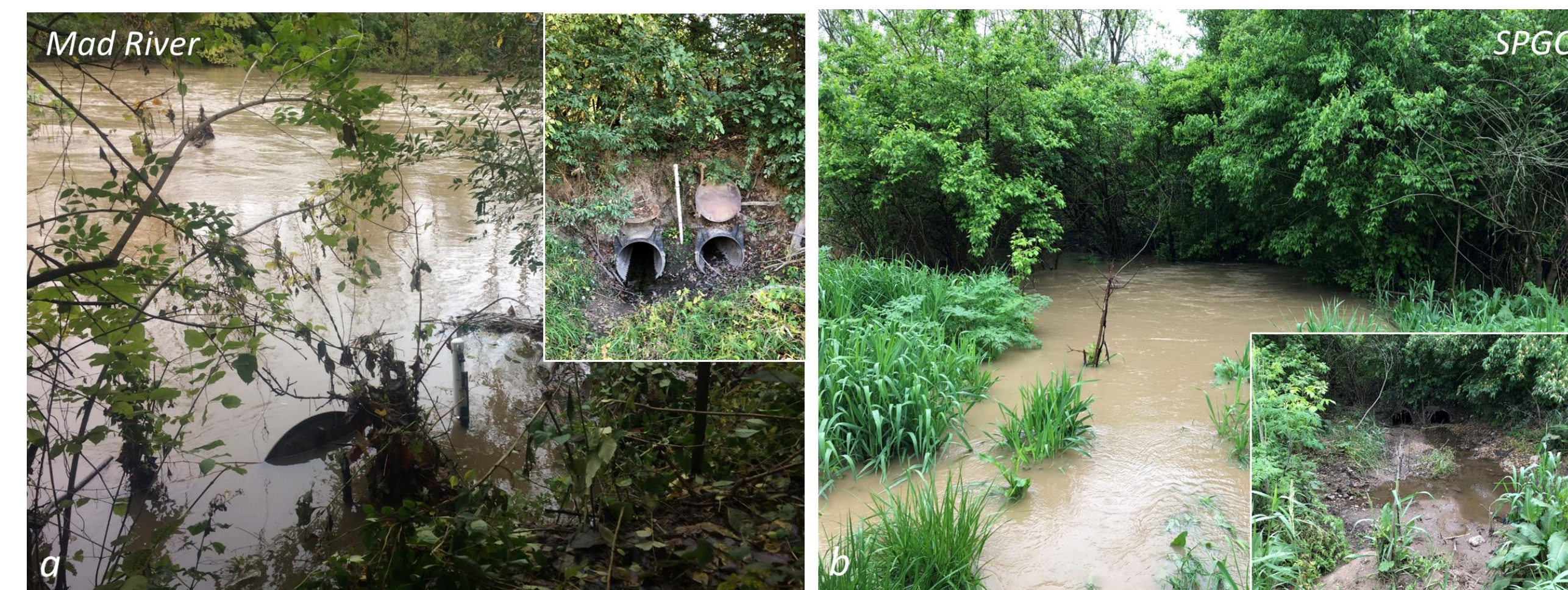
Figure 5. a) Flapper gates on the Mad River side limited flow from Mad River during floods while allowing for drainage of flow from the golf course. The culverts are submerged during the flow event shown. The inset shows the housing for one of the levelloggers during low flow. With the flapper gates open, the Mad River is essentially hydrologically reconnected to its former floodplain. b) Submerged culverts on the former SPGC side would have drained the course during operation but now allow flow onto the course. A second levellogger on the SPGC side is used to measure the difference in head between Mad River and the course.
