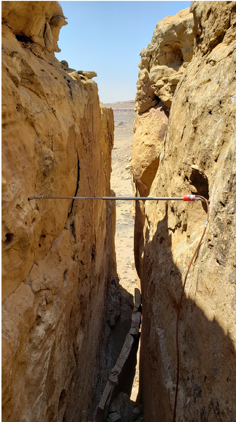
Figure 1. Photograph of a vibrating wire extensometers (crackmeter) in Cliff House Sandstone at Chaco Culture National Historical Park, New Mexico. Crackmeters such as these can be installed across rock fractures ranging from several millimeters to several meters wide. The crackmeters are anchored into the rock with epoxy and then covered with a plastic or aluminum cover to keep the sensor shaded from direct sun and keep any potential snow weight off the sensor. (National Park Service photograph).
