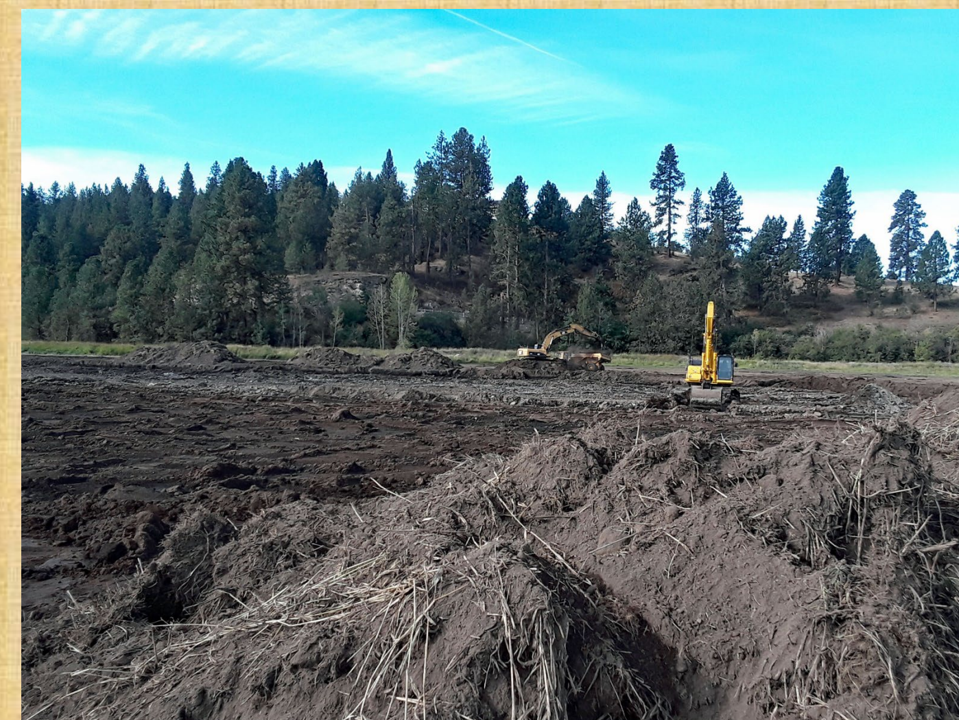
Left: Saltese Flats project site, and Spokane County wetlands restoration project: initial excavation and pre-exposure of Mazama ash deposit.
