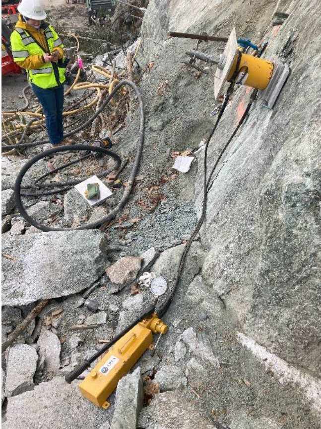
Rock dowel pull testing, Fairlee (Scarptec, 2024)
