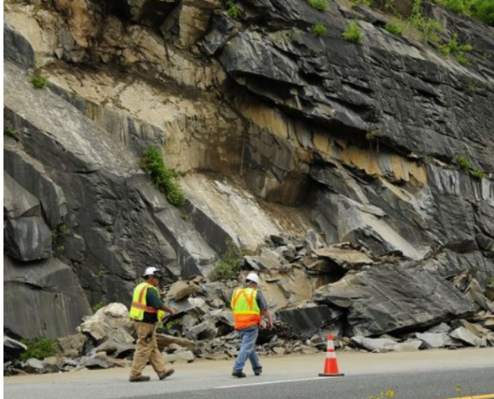
Rockslide I-89 NB, Exit 6, Berlin, July 2012 – note metalimestone bed between phyllite/schist layers (Waits River Fm; VTrans)
