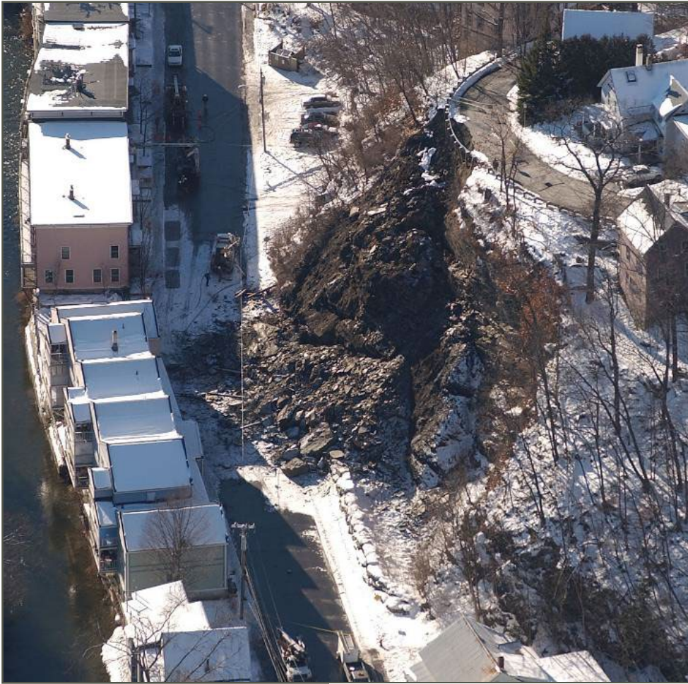
Elm St. Rockslide, Montpelier, December 2005 (VTrans)
