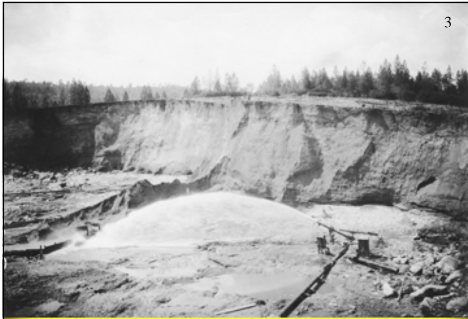
Hydraulic mining at the Esperance Mine, French Corral, California
