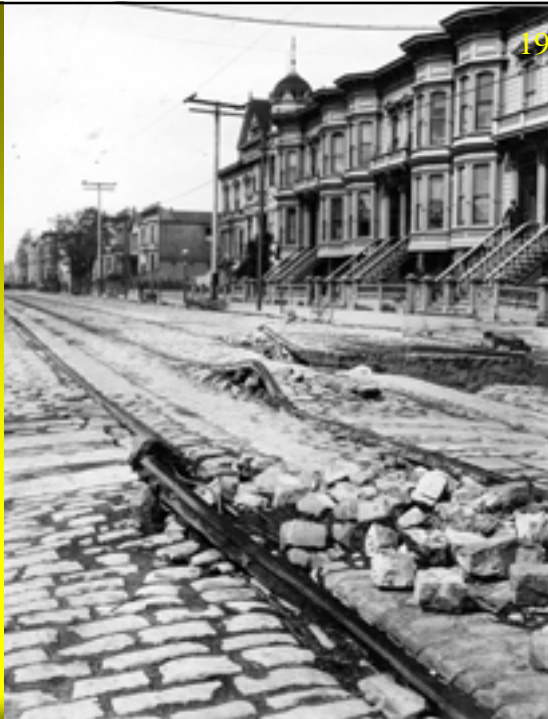
Buckling caused by earth flow, Howard Street, San Francisco, 18 April 1906 USGS Photo Archives, Denver
