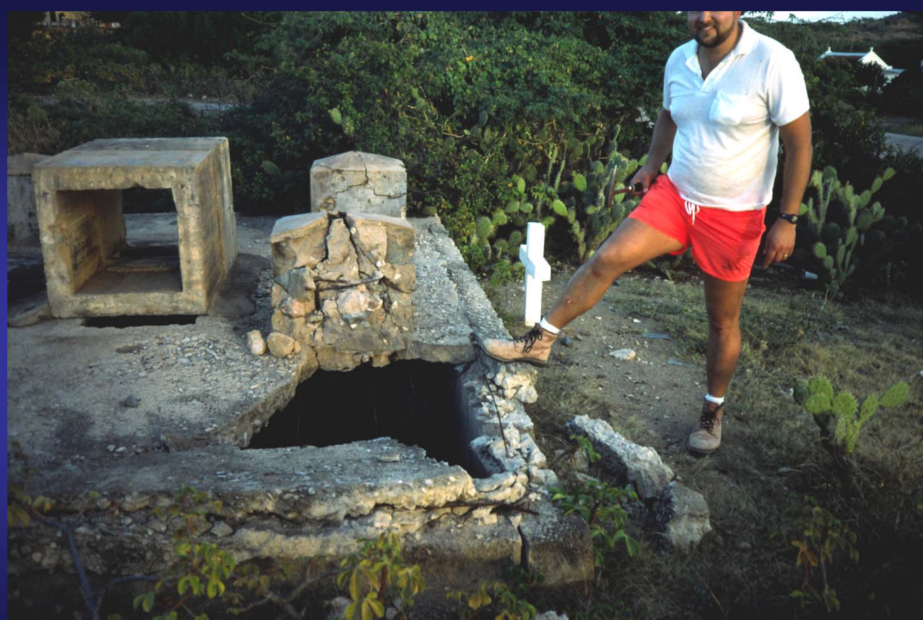
Bob Salna and caved concrete cover for Calabasa shaft, north Aruba -- cross from 1935 death to his right. Near-death experience for Salna and Pride, especially Salna, when the slab gave way as we stepped onto it, a slab that we both were walking around on two days previous. It's 40+ feet down to water (photo by D.E. Pride).
